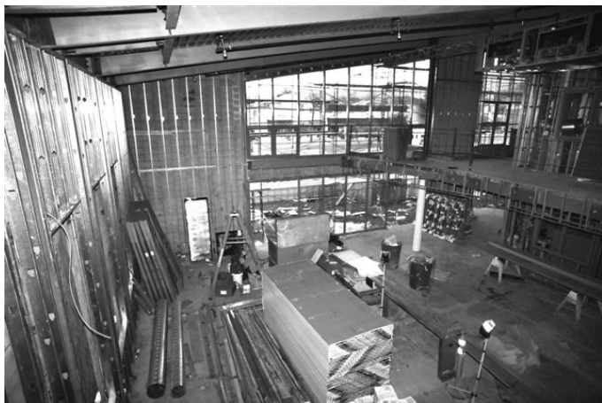
Social hall as viewed from second floor classroom.
