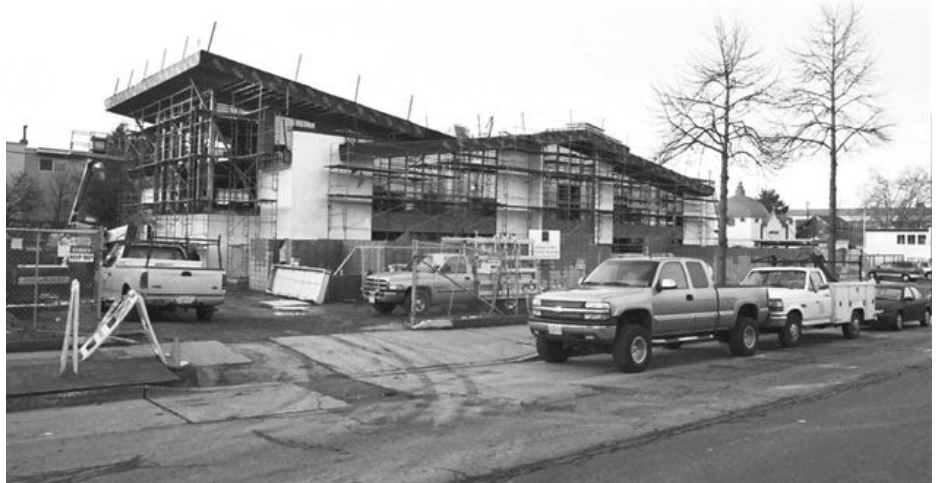
View from University Avenue: the building is now surrounded by scaffolding to allow installation of glazing and exterior finishes.
