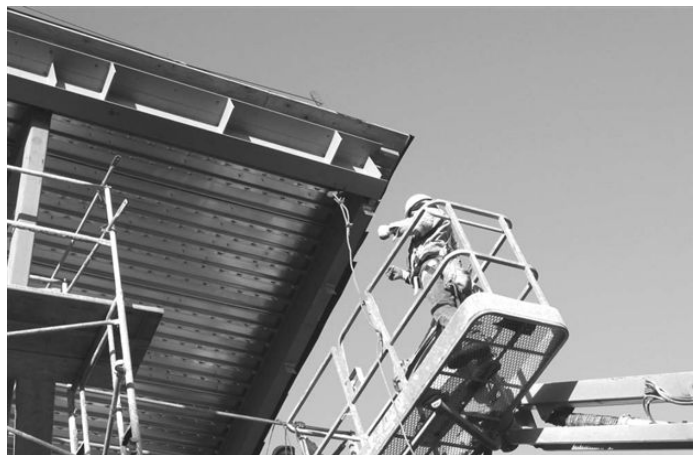
A “cherry picker” elevates these construction workers to the roof eave to complete the soffit installation.
